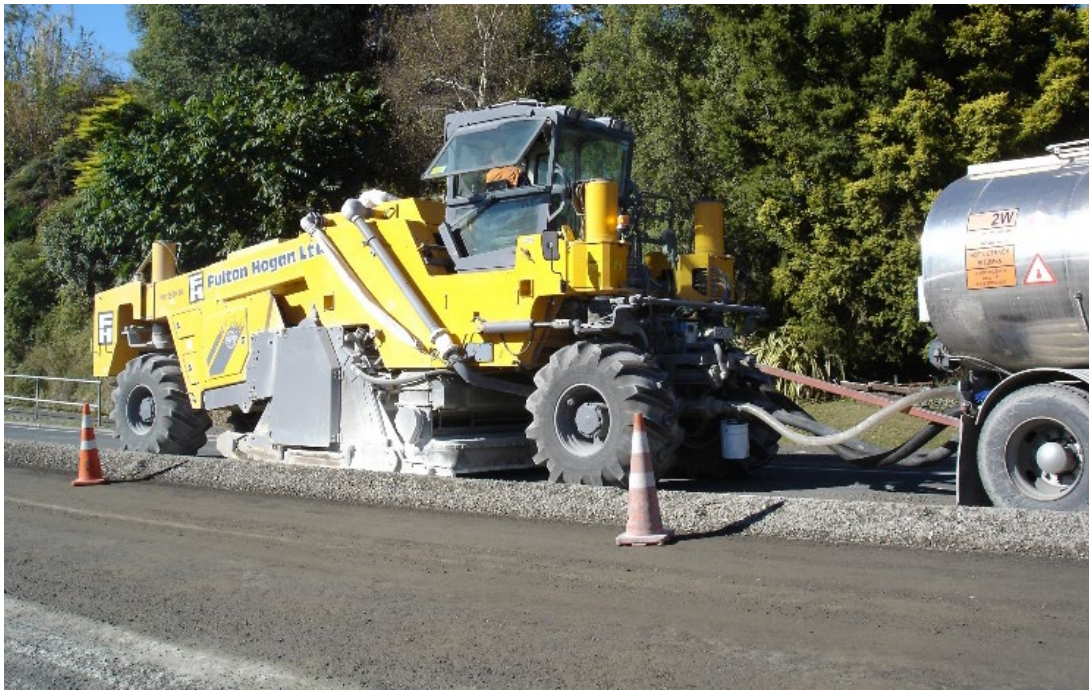
Figure 4.7 Stabilisation of road aggregate to bond particles.
