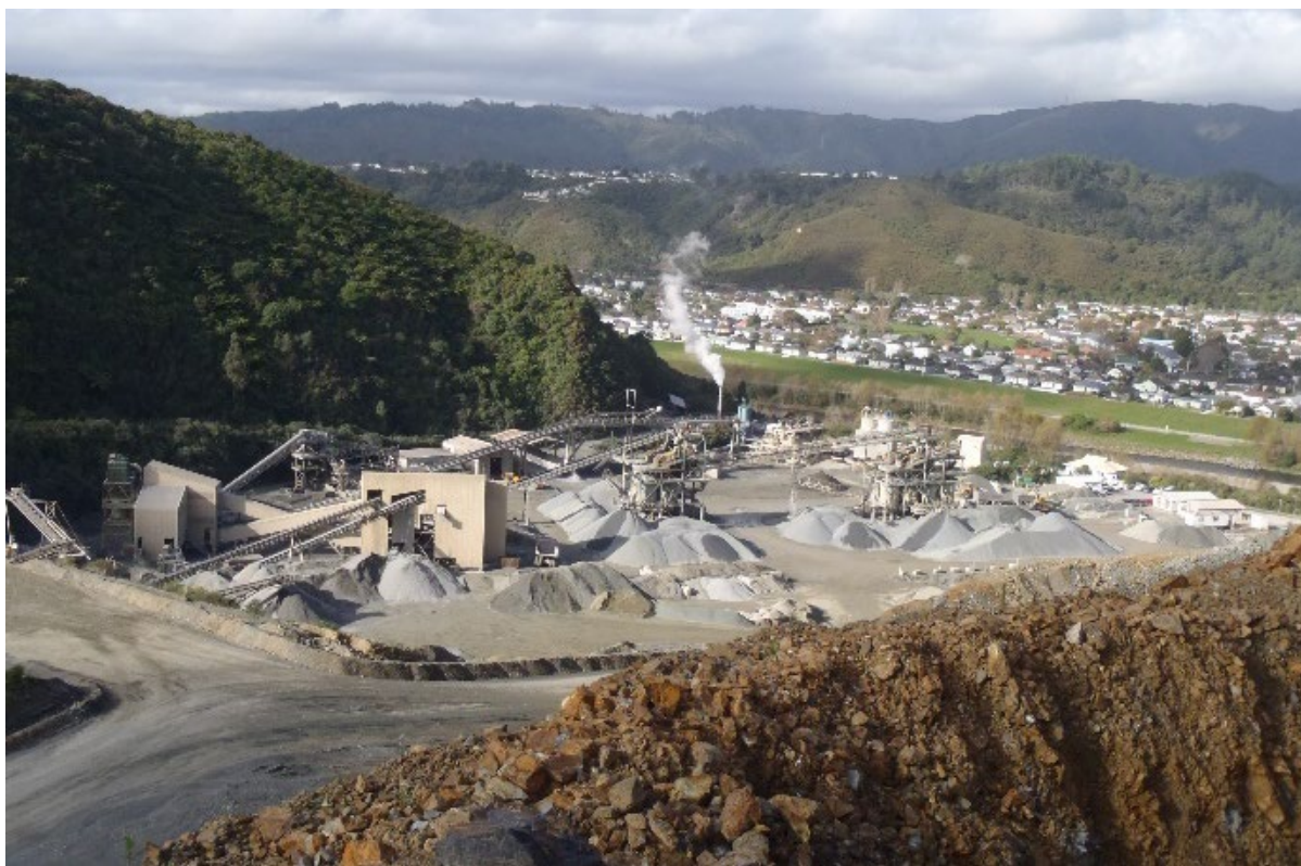
Figure 4.3 Aggregate processing plant at Belmont quarry in Lower Hutt. Greywacke rock is quarried and then crushed and screened into various-sized products.
